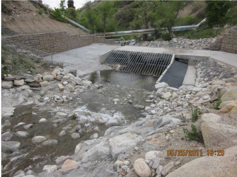
Figure 4-1 Debris Collecting Structure on Big Cottonwood Creek, Salt Lake County, Utah
