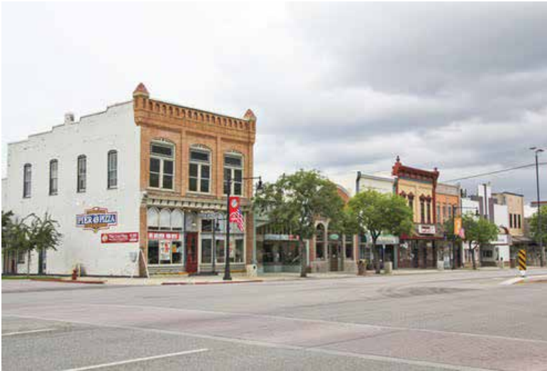
Figure 5.1 Springville received funding through MAG to modify Main Street to revitalize the downtown area.
