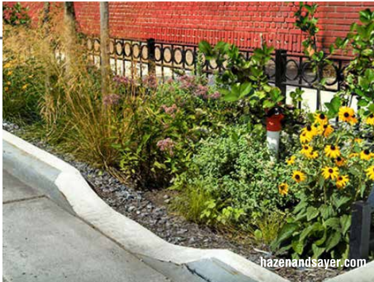
Figure 2.13 Curb cuts at each bump out will allow storm water to flow into the landscape areas.
