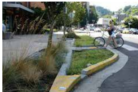
Figure 5. Regularly spaced curb cuts allow storm water to be harvested into landscape bed areas.
