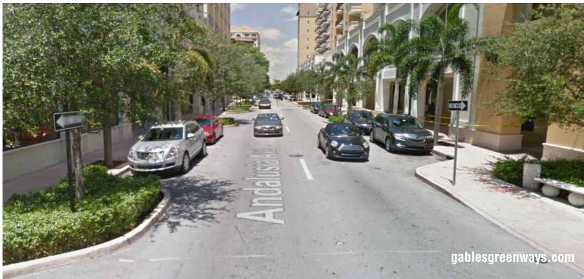
Figure 2.14 Curb bump outs create space for aesthetic landscape design and traffic buffering.
