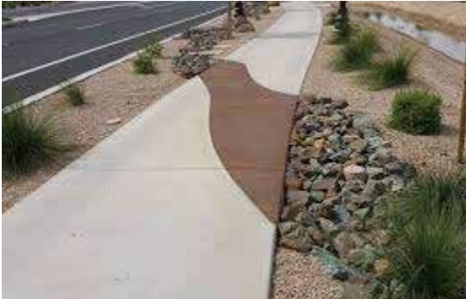
Figure 1. Combination of different concrete finishes. By adding an exposed aggregate ribbon the hardscape picks up the river theme throughout the project.
