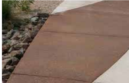
Figure 2. Adding a stain or Natina concrete color treatment adds additional accentuation to the hardscape.
