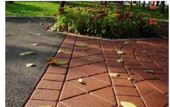
Figure 6. Colored and stamped asphalt used for crosswalks offer a visual delineation from the main roadway traffic.
