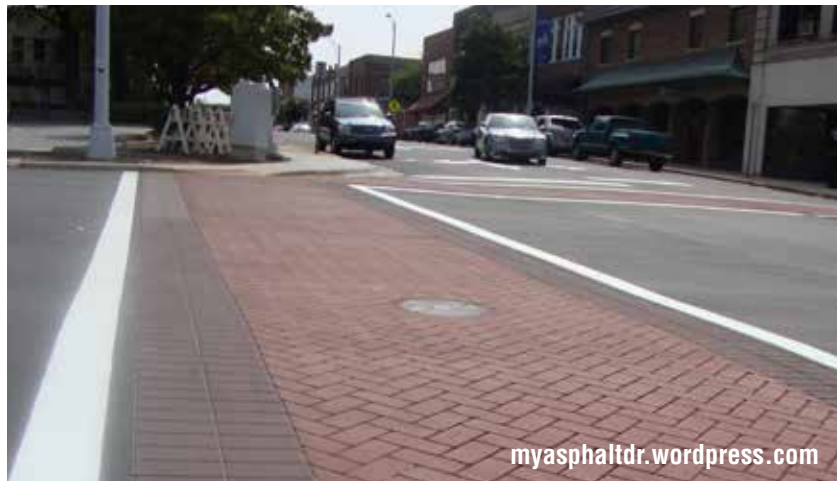
Top to Bottom: Figure 2.11 To create a more visually appealing corridor, a variety of concrete finishes are proposed to represent a flowing river leading the visitor through the space. Figure 2.12 Stamped asphalt or in-laid reflective tape, such as those pictured above, will help improve the visibility of crosswalks.
